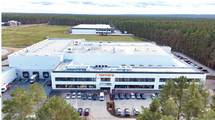
Figure 5: State-of-the-art manufacturing facility, hosting cleanrooms compliant with BREEAM recommendations.
